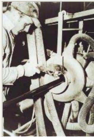
Fig. 4. Pipe emerges from the "octopus" air blower-coating chamber, used at Banister's Warren, Ohio, FBE pipe-coating plant, in the early 1960s. Photo courtesy Rupert F. Strobel, 3M Co.
