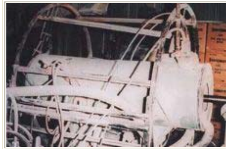
Fig. 5. H.C. Price was the first company to apply FBE to pipe by electrostatic spray, using a Ransburg electrostatic spray system. Photo courtesy Rupert F. Strobel, 3M Co.
