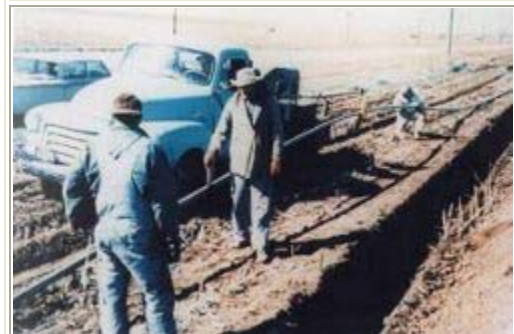
Fig. 2. Crews install the first pipeline coated with 3M's Scotchkote 101 for
