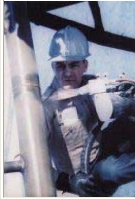
Fig. 3. In an attempt to respond to pipeline contractor needs, in the early 1960s 3M worked with a Minneapolis- based welding equipment company to design and build equipment to flame-spray epoxy powder on weld joints. Photo courtesy Rupert F. Strobel, 3M Co.
