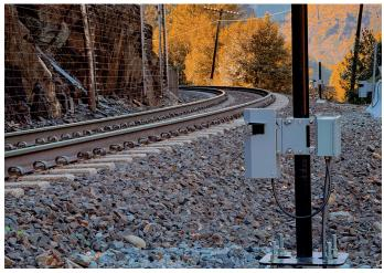
Real-world trials with leading railway companies have demonstrated the reliability of L.B. Foster's Rockfall Monitoring. The system successfully detected every rockfall event during testing. It also significantly enhances operational efficiency while lowering costs by reducing maintenance callouts by over 90% and cutting slow order time by 98.5%.
