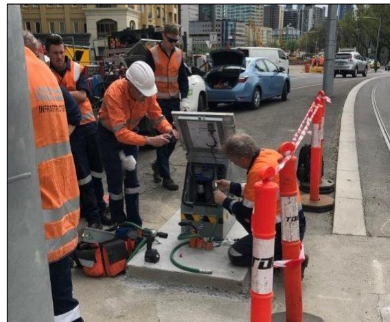
Figure 15. Day 4 of Inbound Track TOR unit installation
