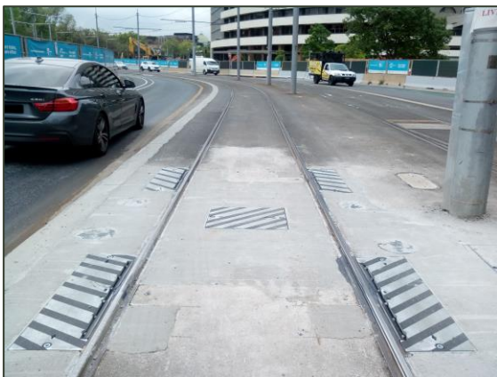
Figure 16. St. Kilda Road Outbound Track TOR Site
