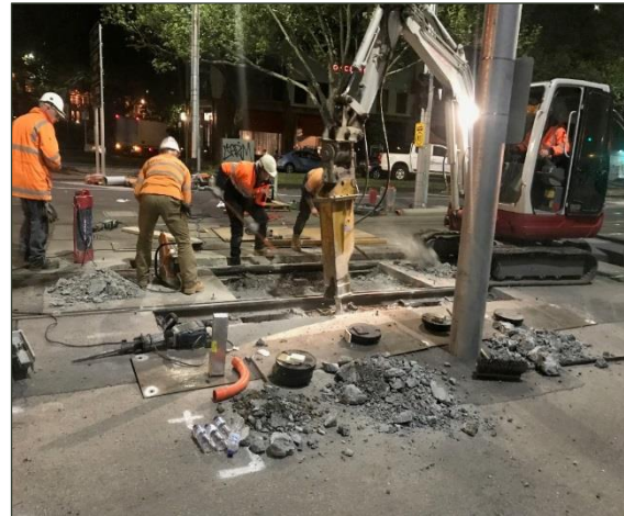
Figure 12. Day 1 of Inbound Track TOR unit installation
