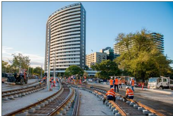
Figure 1. Domain Precinct Temporary Tram Works
