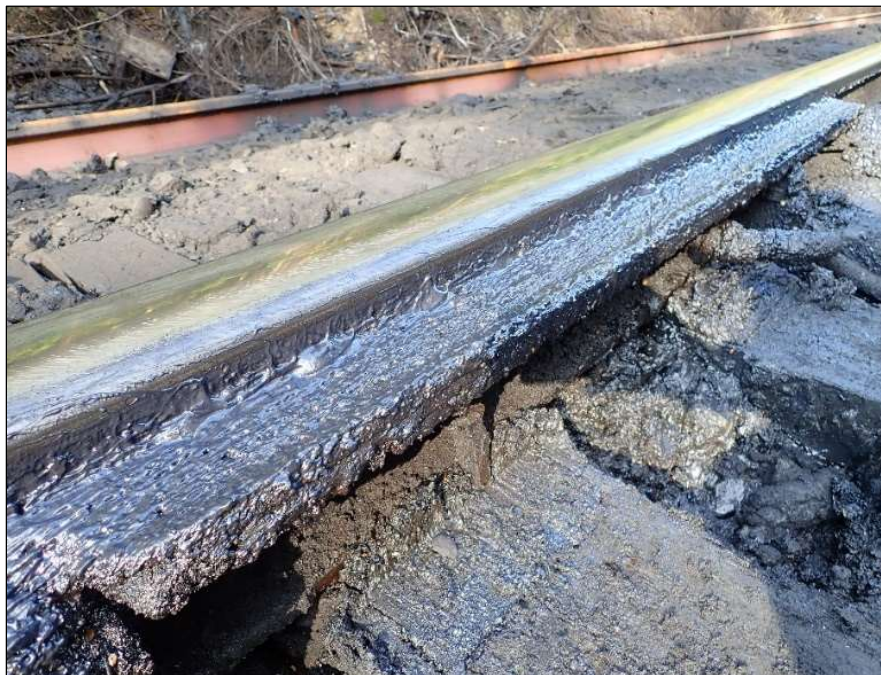
FIGURE 1: Winter grade traditional petroleum-based grease applied in warm summer temperatures, resulting in low viscosity and fling-off.
