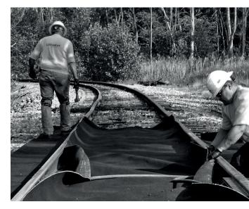
At trackside FM system sites, **GTPlus75** track mats are placed over the ties, protecting the soil and ballast from contamination.
