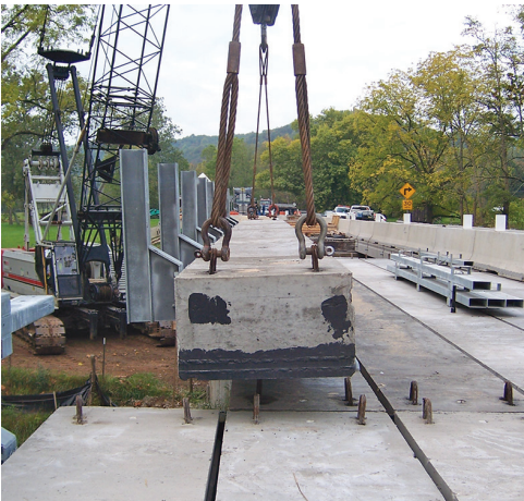
BRIDGE BOX BEAMS
