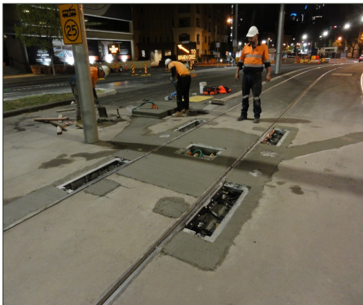
Figure 14. Day 3 of Inbound Track TOR unit installation
