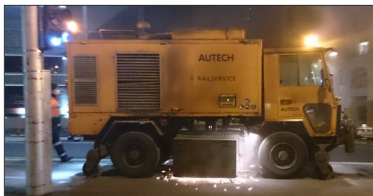
Figure 5. Rail Grinder Truck on St. Kilda Road
