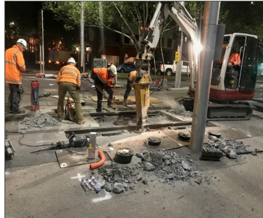
Figure 12. Day 1 of Inbound Track TOR unit installation
