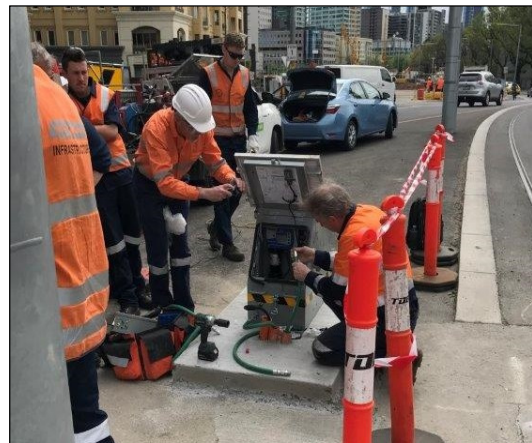
Figure 15. Day 4 of Inbound Track TOR unit installation
