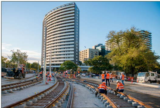
Figure 1. Domain Precinct Temporary Tram Works
