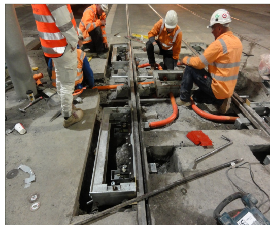
Figure 13. Day 2 of Inbound Track TOR unit installation
