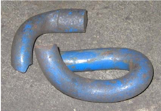
Figure 1 Example of typical broken clip
