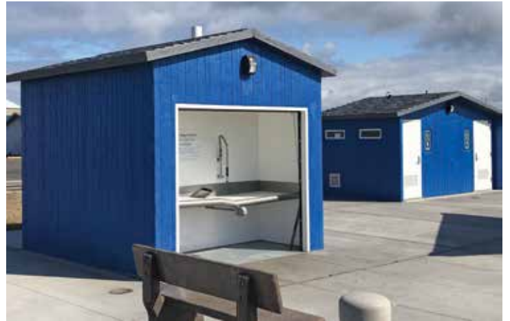
Flush restroom and fish cleaning station
