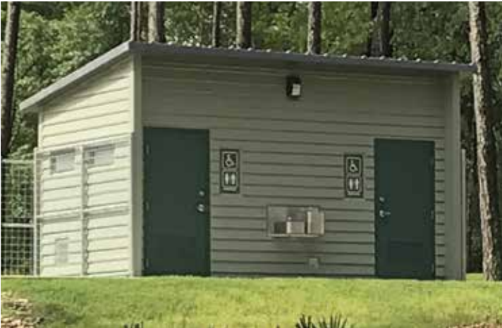
Flush restroom with custom roof pitch
