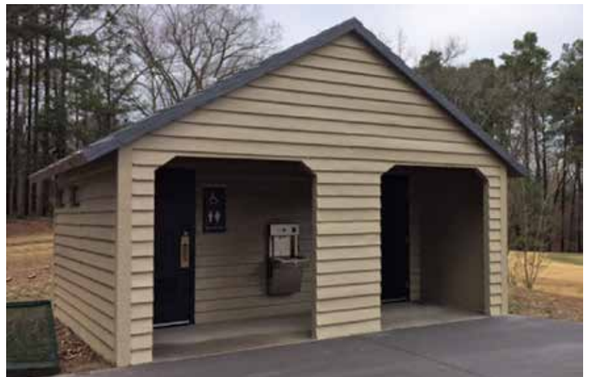
Flush restroom with golf cart shelter
