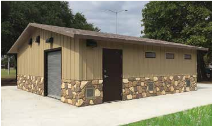
Flush restroom/concession with custom roll up door
