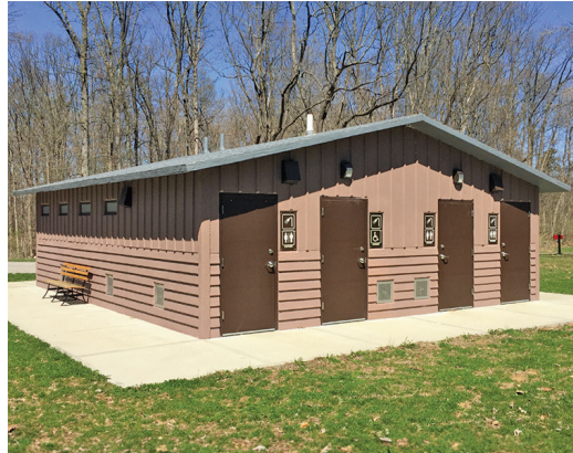
Cheyenne - 26' x 30' Two Multiuser Fully Accessible Restrooms with Four Separate Shower Rooms
